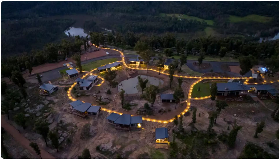
📷 A connecting path at the Kangaroo Valley Bush Retreat is illuminated by bollard lights, creating a spectacular appearance. Picture supplied.
